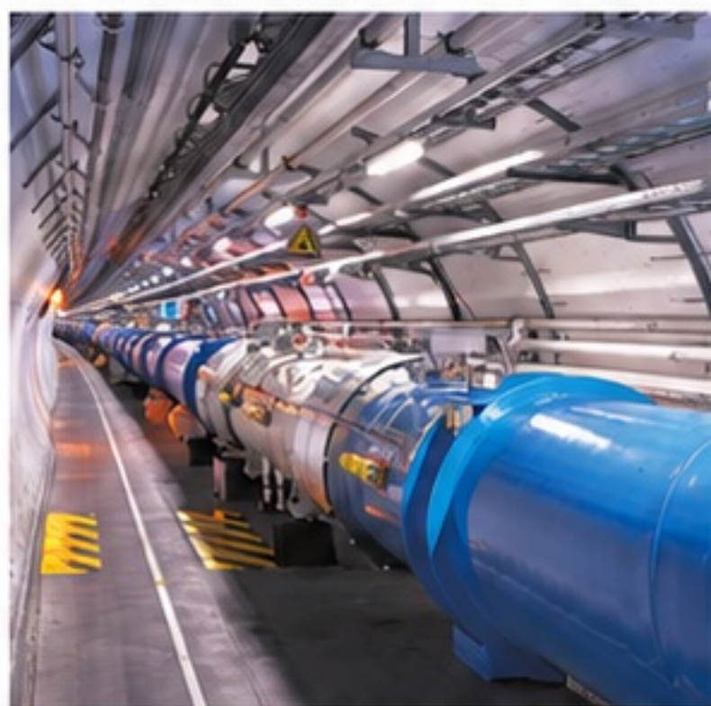
A view of the LHC tunnel MAXIMILIEN BRICE/CERN
